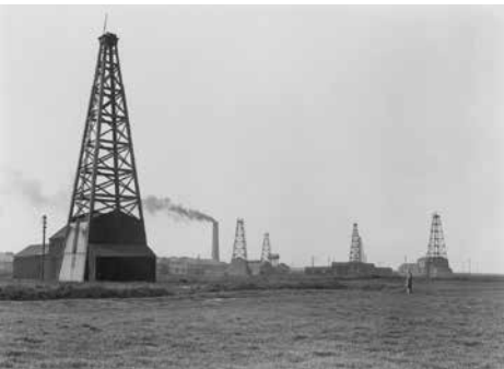
Drilling Rig near Greatham (IH)
