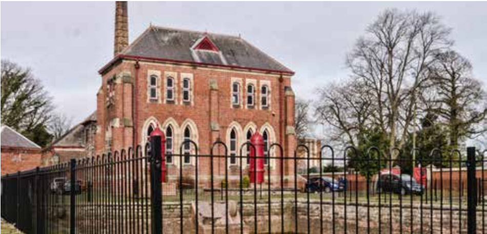
Tees Cottage Pumping Station (PG)
