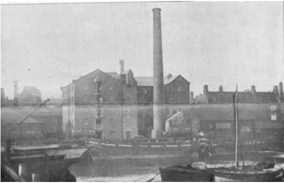
1840 Flour Mill on Stockton Riverside c1905
