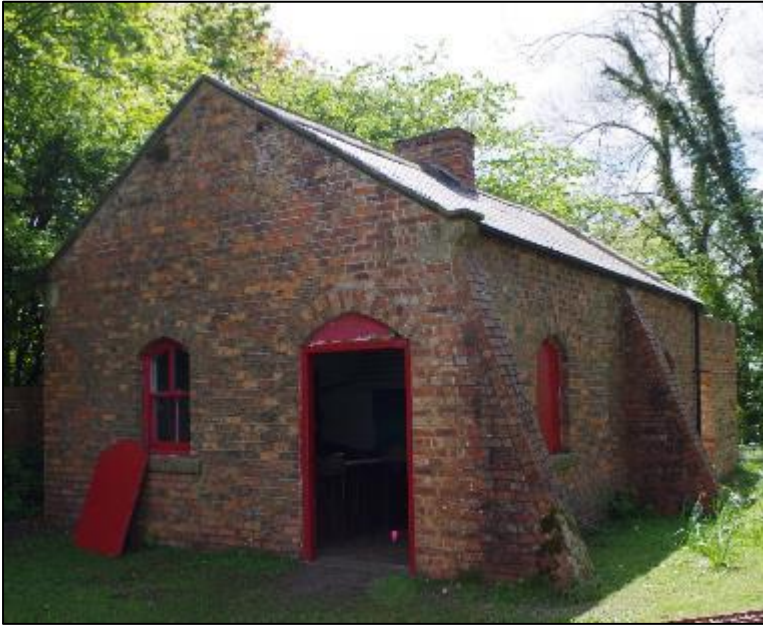
Figure 26. Blacksmith's Shop, north and west elevations and interior. The building was authorised by company minute of 22/9/1853 but seemingly not built till after the 1 st Edition OS survey of 1855.
