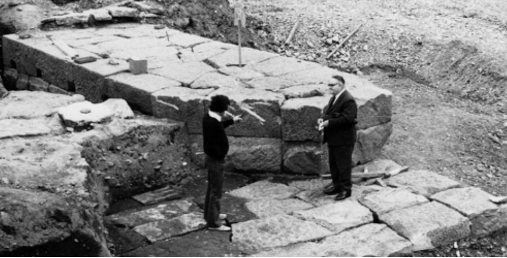
South bridge abutment during excavation (DCC)
