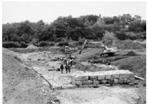
Bridge foundations being uncovered in 1972 (DCC)
